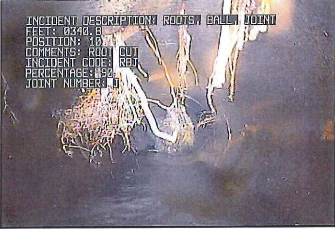
RBJ - Roots, Ball, Joint @ 340.8 ft. root cut
