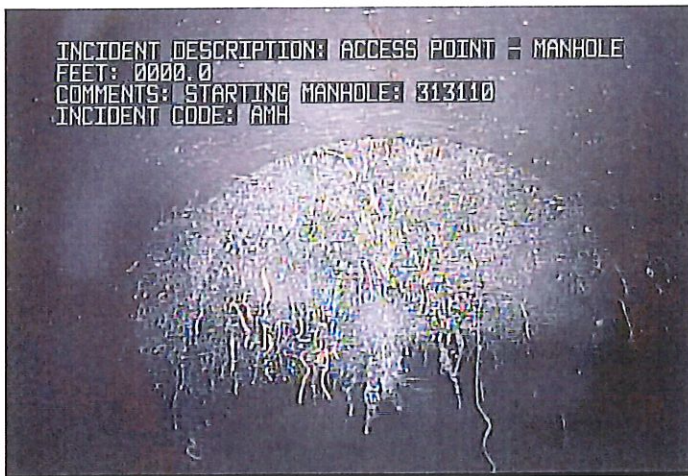
AMH - Access Point - Manhole @ 0.0 ft. Starting Manhole: 313110
